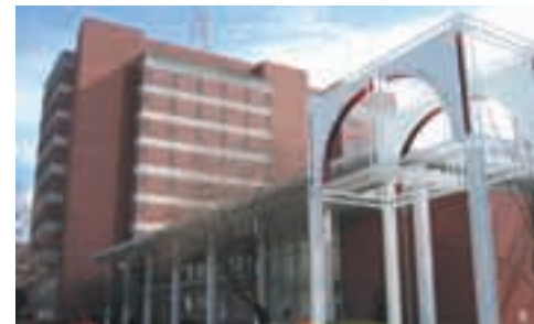
College of Engineering at North Carolina State University
